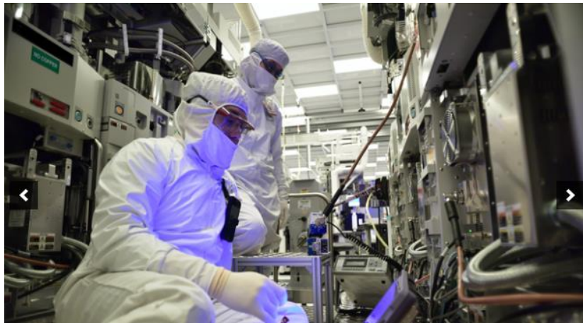
Figure 3: A typical installation project environment: production and cleanroom facilities at work in Hillsboro, Oregon (credit: Intel Corporation newsroom).
